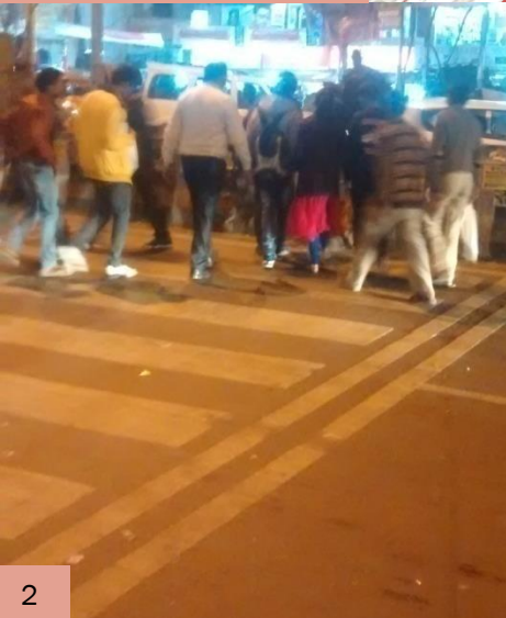
2 No sync between width of zebra crossing and opening of median
