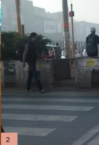
2 No sync between width of zebra crossing and opening of median
