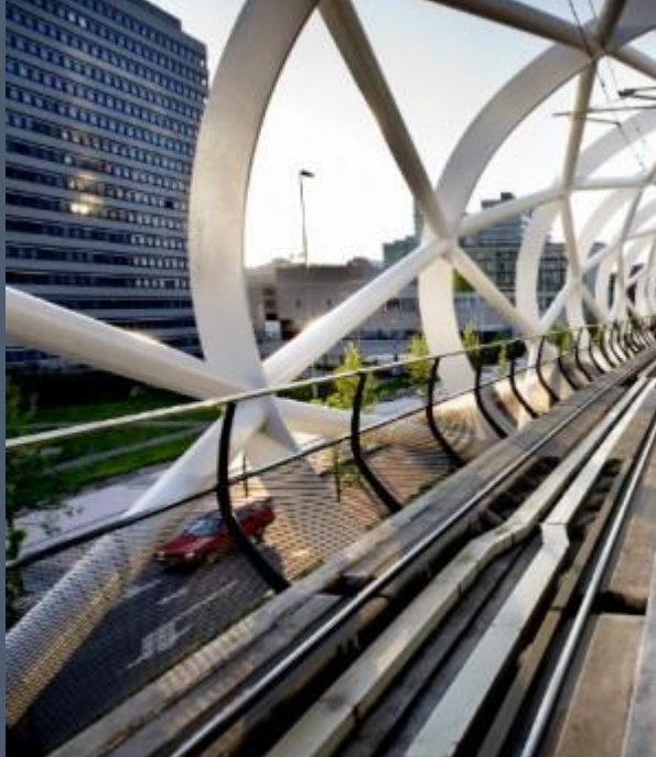
Hague Beatrixkwartier Light-rail station
