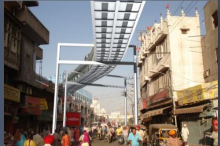
Double Column Support Guide way as portal frame
